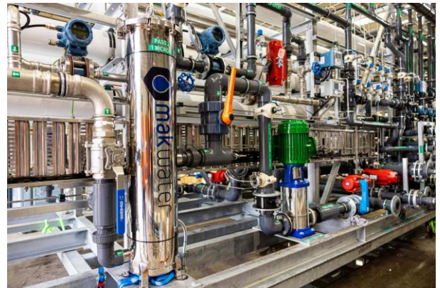
Skid-mounted stainless steel 316 (SS 316) RO plant
